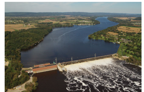
Prairie du Sac Hydroelectric Project
